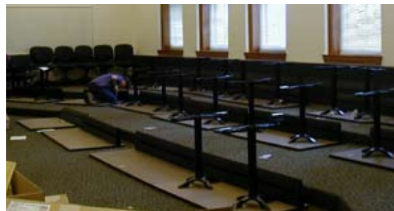
A worker installs tables in the computer classroom.
