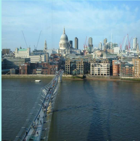
Figure 3. London's Millenium Suspension Footbridge over the Thames.
